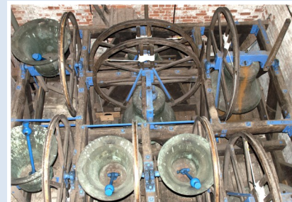
Bell in the up position, ready to be rung
